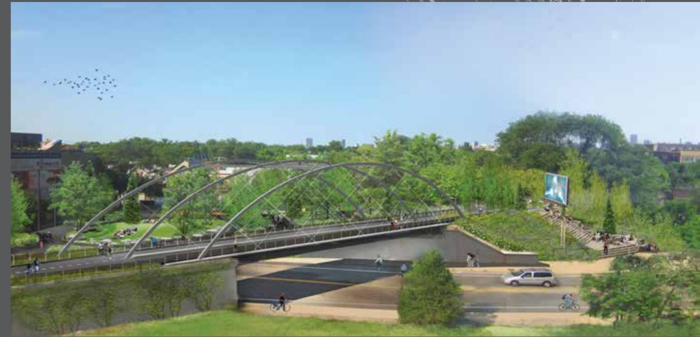
BRIDGE, BILLBOARD AND STAIR AT MILWAUKEE AVENUE
